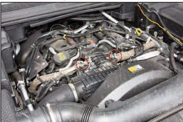
EGR pipe clamps
